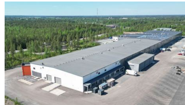
New production facility for sheet metal mechanics opened in Oulainen, Finland
