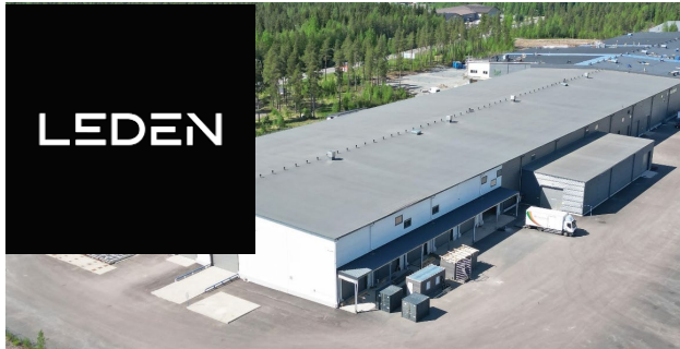
New state-of-the-art sheet metal factory in Oulainen.
