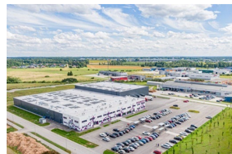
HANZA's new building for complex assembly, pictured left.
