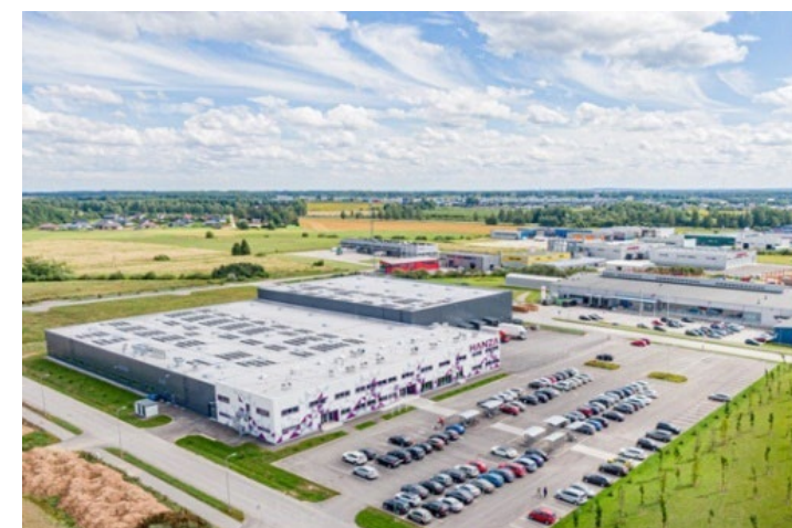
HANZA's new building for complex assembly, left in the picture.
